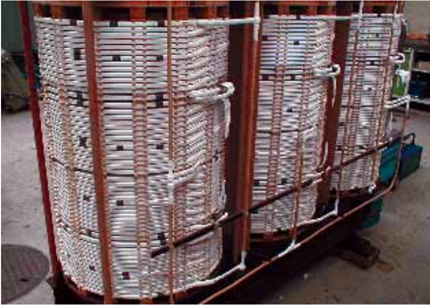
Illustrations show Transformer before (upper right photo) and after retrofit using NOMEX® Thermal Technology for protective insulation (left photo).
